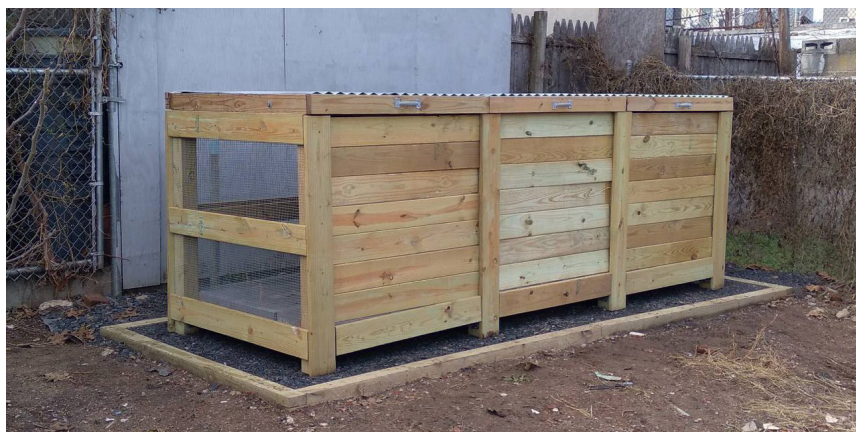
Photo: Side profile of a compost bin system, showing the hardware cloth and pavers at the bottom of the bins.
